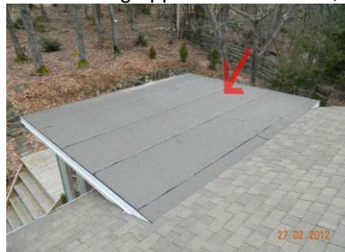
roof covering appears serviceable
