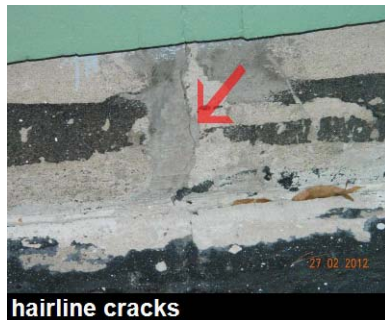
hairline cracks
