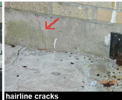
hairline cracks
